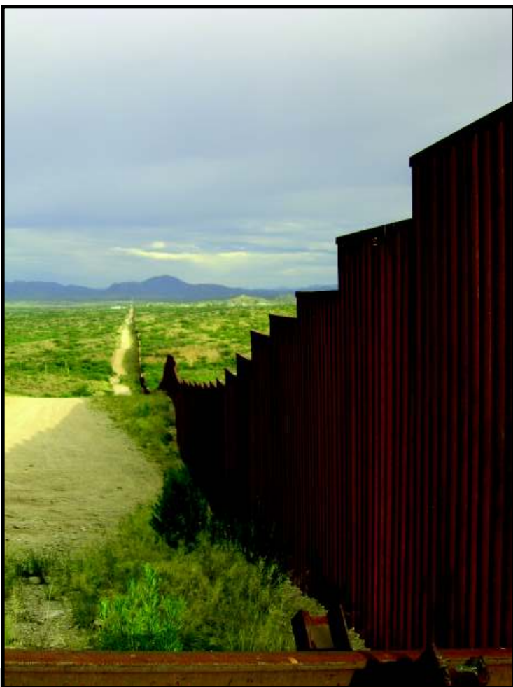
The border fence in Arizona comes to an abrupt end directly to the right of this photo. (Photo: Jamie Way)
