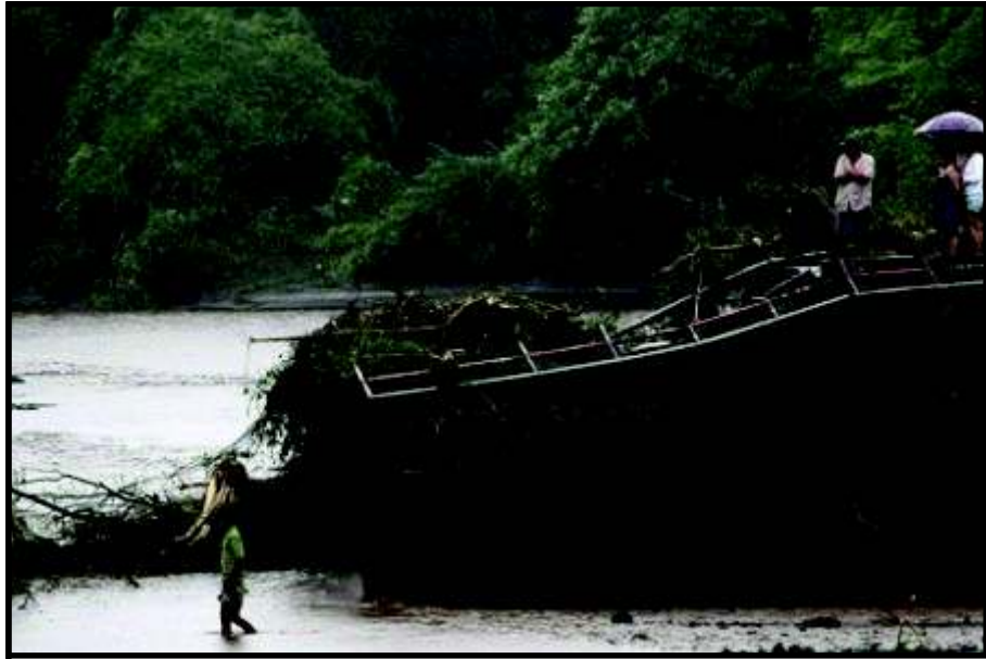
A bridge damaged by heavy rain in Quezalguaque, Nicaragua. (Photo: PressTV)
